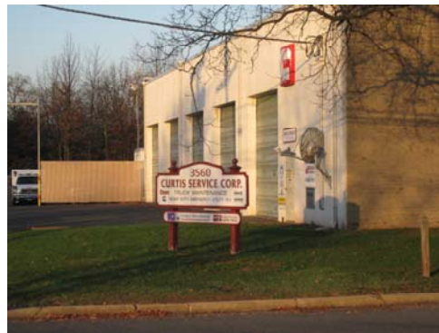
6 South Plainfield, NJ
